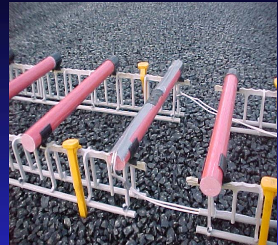
Close-up of instrumented FRP dowel bars
