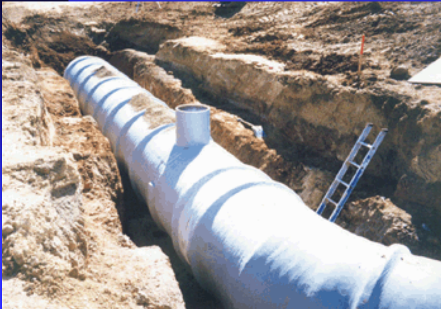
FRP Pipes for Sewerage Works, Bolivar Project, Australia
